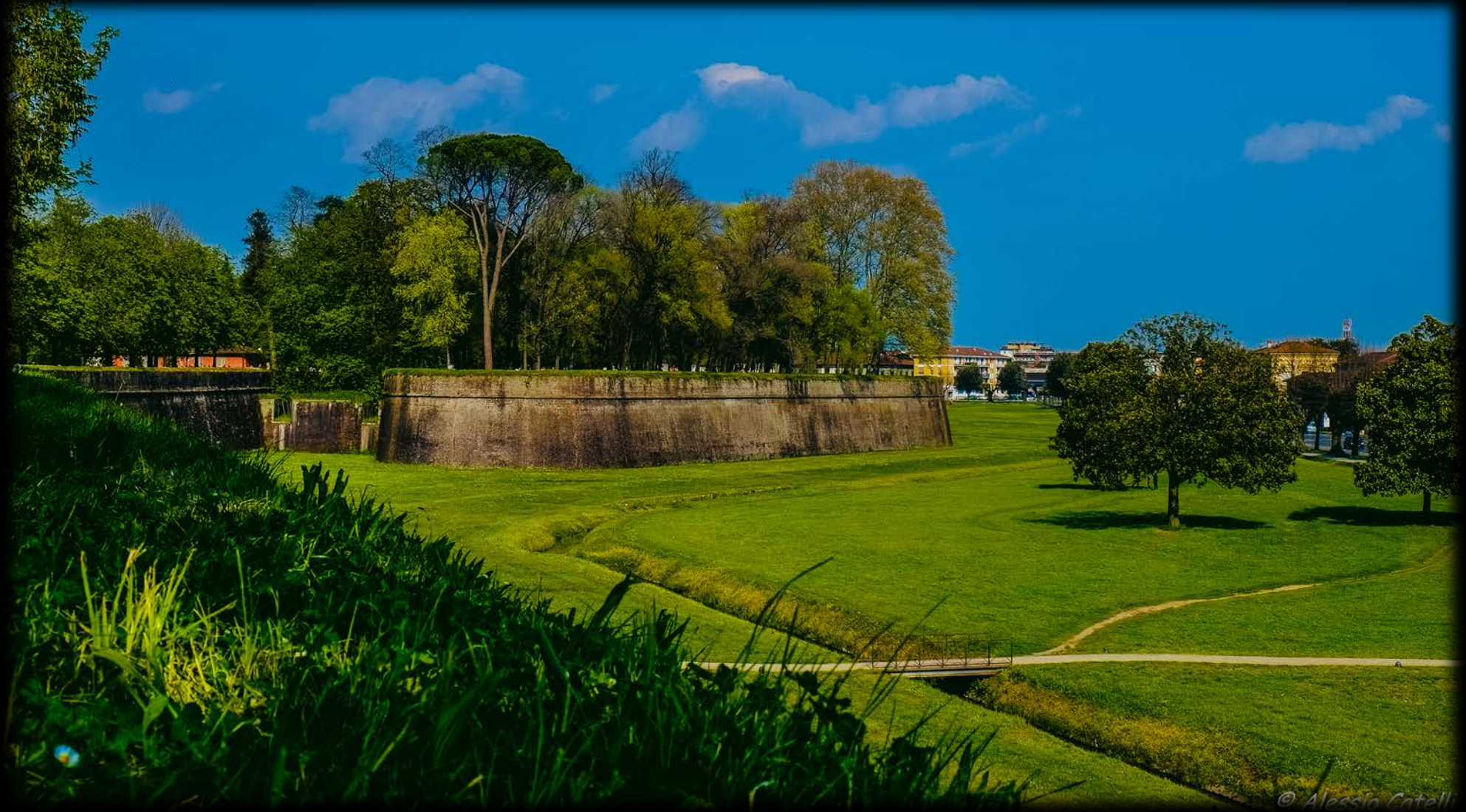
Lucca, The Walls, 16 th century
