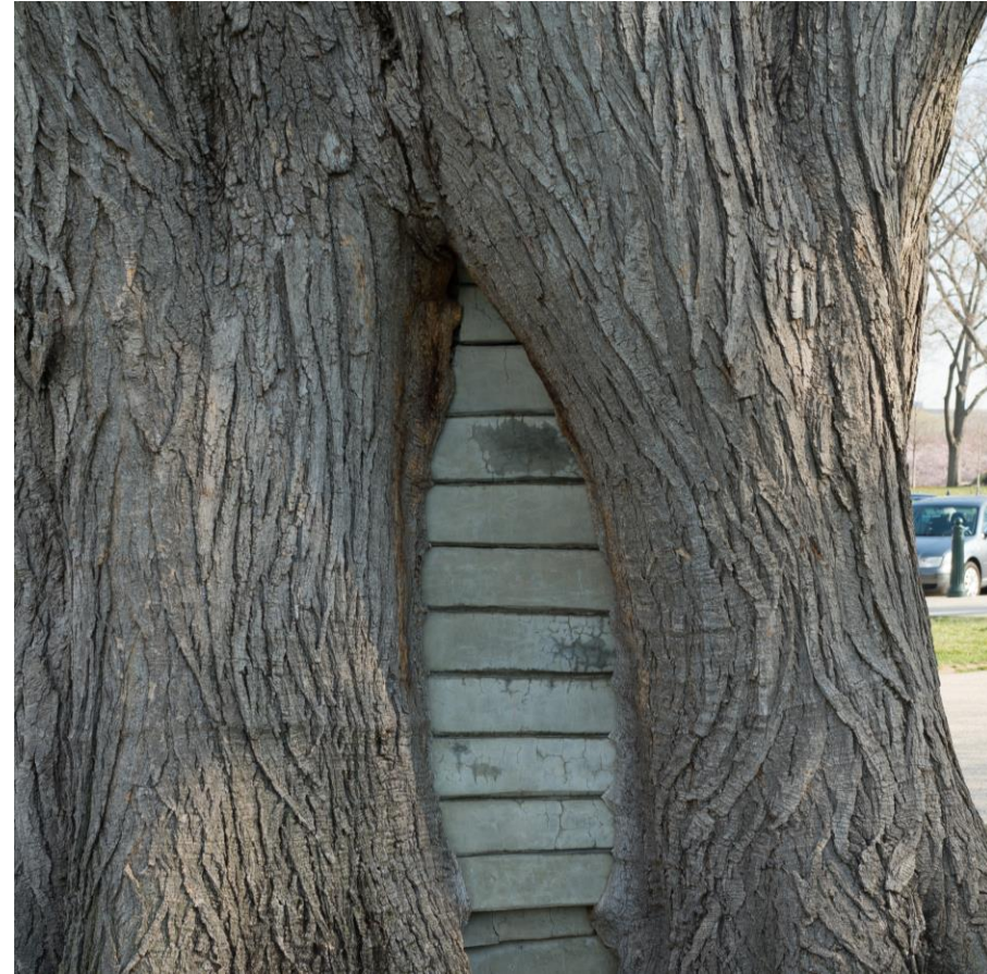
Historic arboriculture: concrete-filled cavity on Olmsted Styphnolobium
