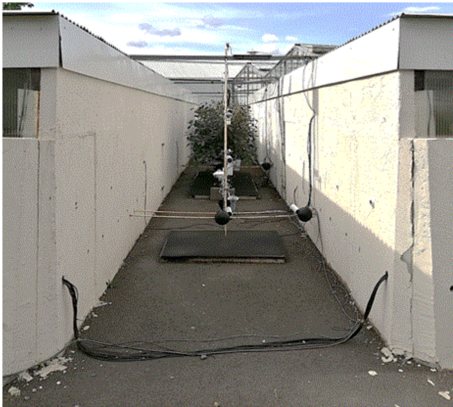
South view of the canyon street at 1/5 th scale built at Institut Agro in Angers, France, on June 23, 2022 (© D. Canonne).
